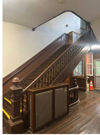
Original Wood Stair
