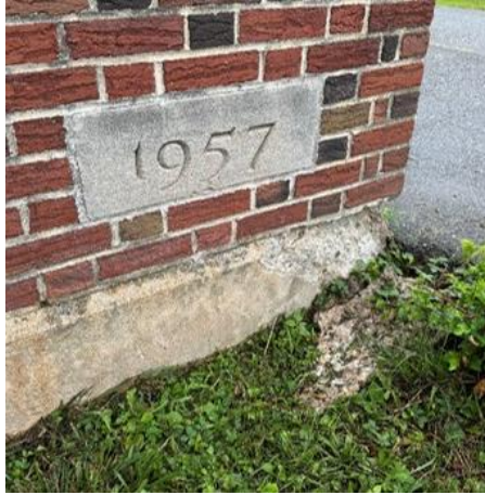
Masonry Spalling
