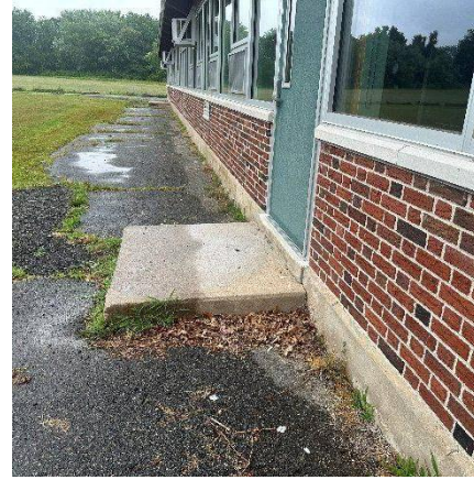
Sidewalk Cracking
