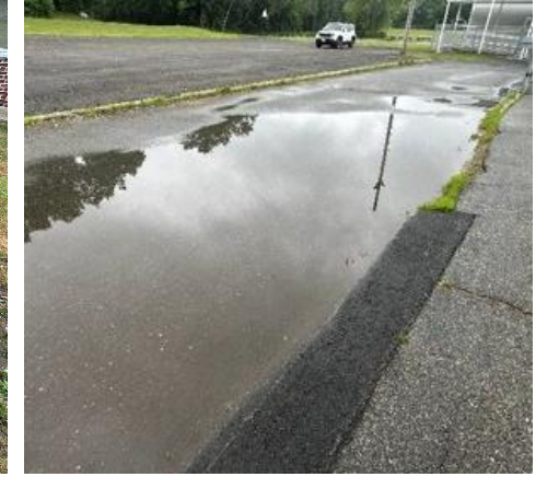
Drainage Ponding
